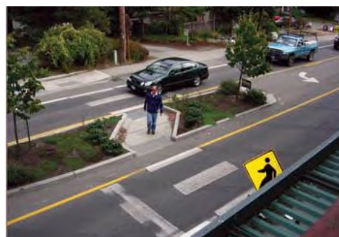
Crossing islands provide refuge for people crossing the street and enable them to deal with only one direction of traffic at a time.
