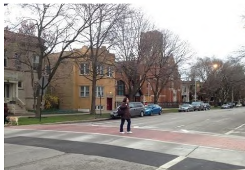
Raised crosswalks can enhance the visibility of pedestrians crossing a street and also help slow vehicle speeds when approaching the crossing.
