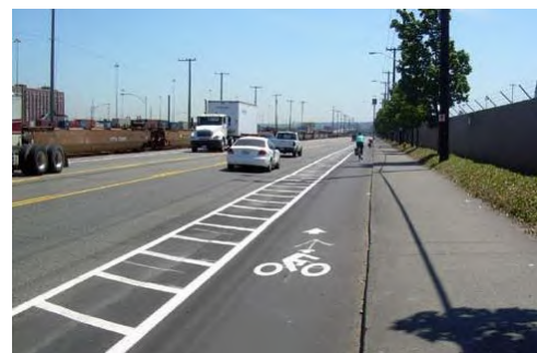
Although integrated into the street surface, buffered bicycle lanes improve bicyclist's comfort by creating a greater separation from motor vehicles.
