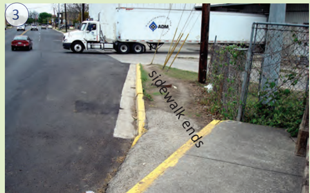
Sidewalk ends at bridge leaving pedestrian in dirt with little refuge from traffic.
