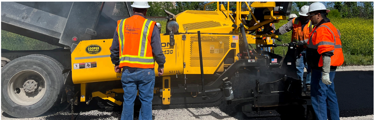
City work crews lay down hot mix asphalt on Church Hill Drive as part of a Mill & Overlay project.
