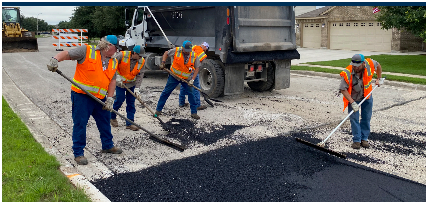
City of New Braunfels Public Works employees spread asphalt while working on a Mill & Overlay project on a portion of Creekview Way.
