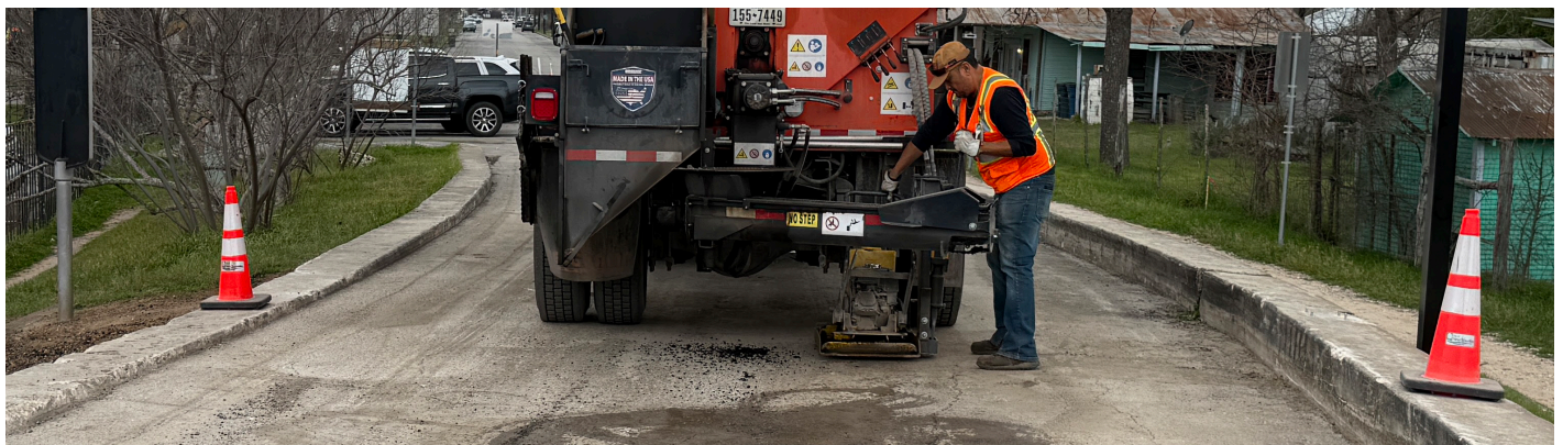
A City of New Braunfels employee finishes patching a portion of Faust Street using hot mix asphalt.
