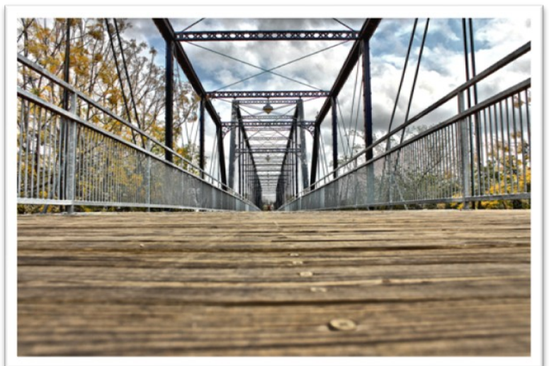
Faust Street Bridge
