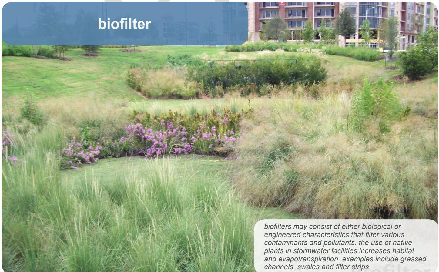
biofilters may consist of either biological or engineered characteristics that filter various contaminants and pollutants. the use of native plants in stormwater facilities increases habitat and evapotranspiration. examples include grassed channels, swales and filter strips
