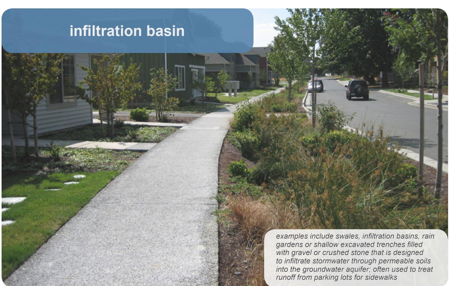
examples include swales, infiltration basins, rain gardens or shallow excavated trenches filled with gravel or crushed stone that is designed to infiltrate stormwater through permeable soils into the groundwater aquifer; often used to treat runoff from parking lots for sidewalks
